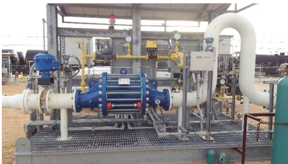
Figure 4. Example of a Paradox USCG-approved in-line detonation flame arrester shown in the author's 2013 technical paper. [1]
